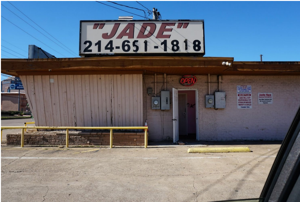
Figure 8. A permanently closed red-light district IMB in a windowless, stand-alone building.
